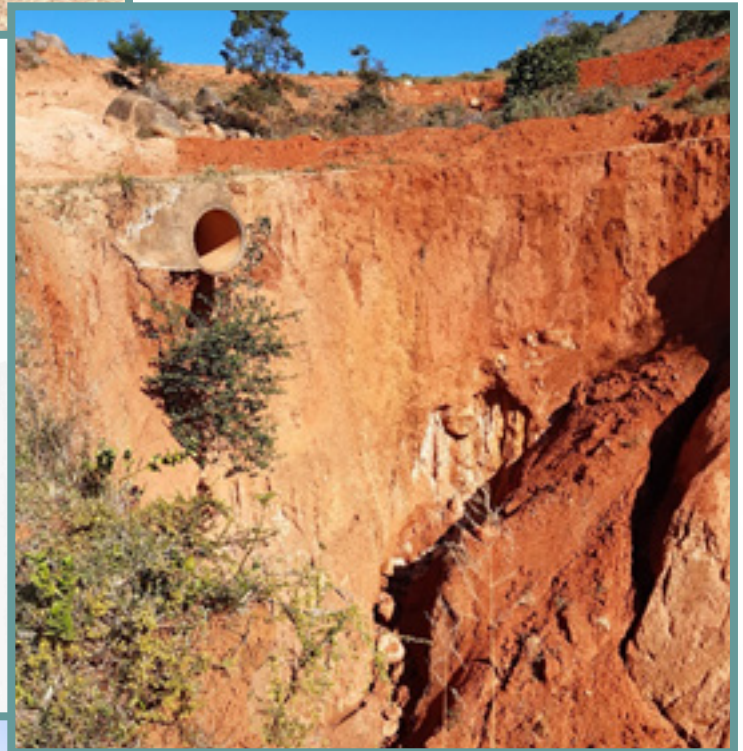
A series of photographs of the gully system in the Sigcineni area threatening the road system (note the road culvert). The rehabilitation is being undertaken by Dept of Public Works, together with EEA/EEF, World Vision , GEP and the community.
