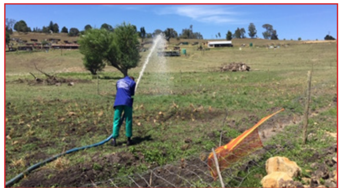
A rehabilitated section of the pipeline (slightly greener) being irrigated to ensure that the seedlings take root during a dry period
